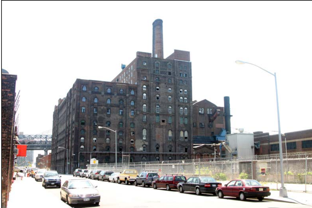
South 2 nd Street facade, view from north Photo: Carl Forster
