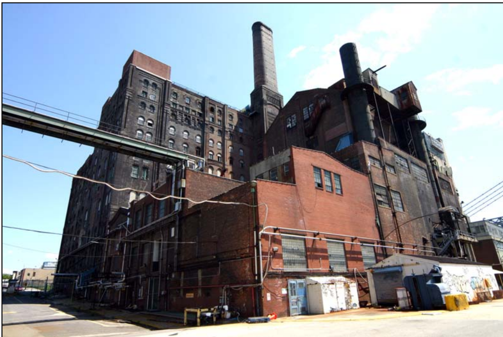
South 2 nd Street and west facade, view from northwest Photo: Carl Forster
