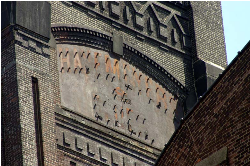
Metal sign, west façade, near roof Photo: Carl Forster
