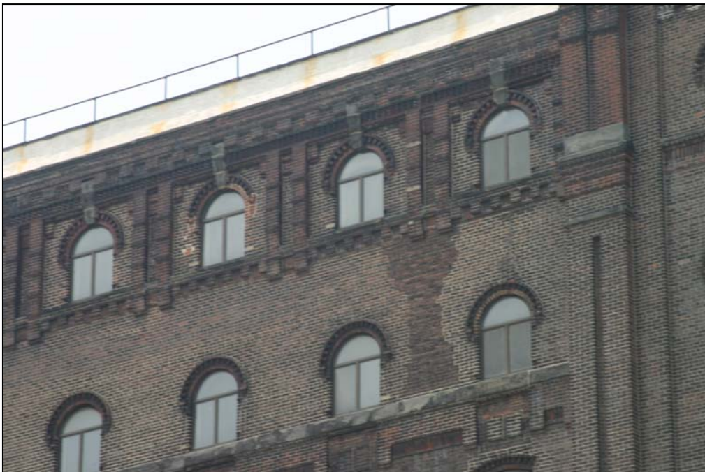
West facade, upper stories Photo: Carl Forster
